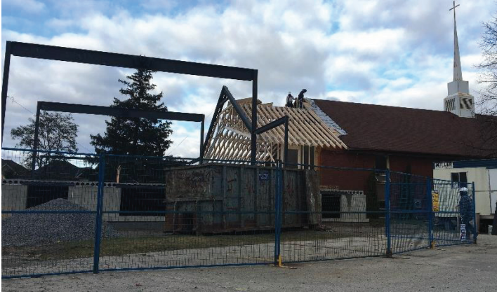
Extending the roof to meet up with the new addition
